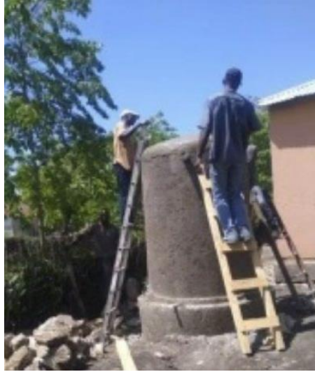
Building a rainwater cistern
